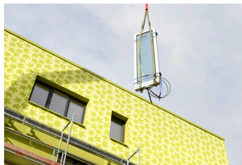
Fig. 21: Mounting a PBR element, March 2013
